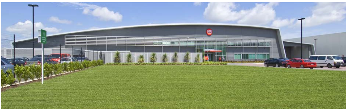
Key customer, New Zealand Post Group, occupies four facilities at Highbrook, including the mail sort centre, shown above.
