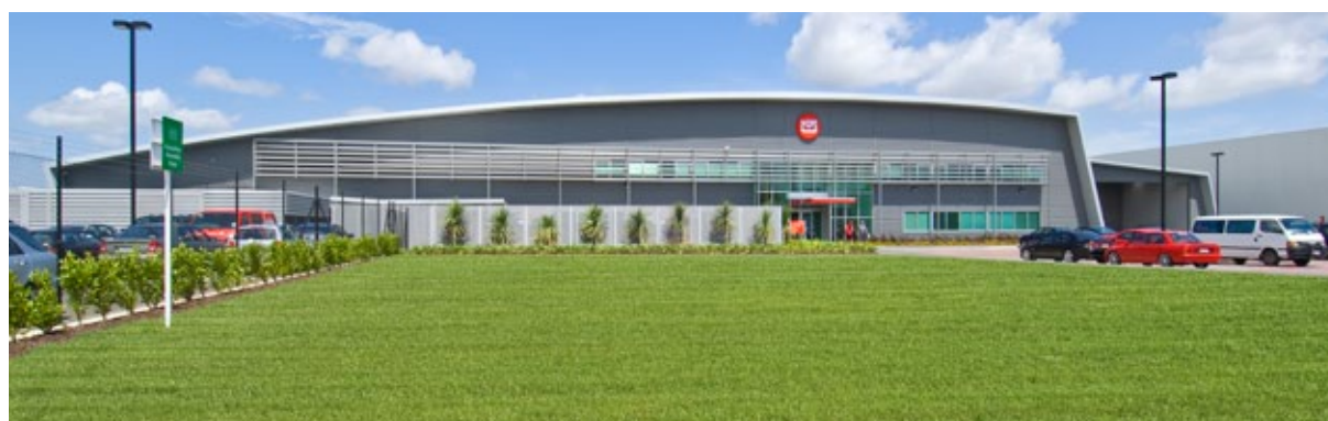
Key customer, New Zealand Post Group, occupies four facilities at Highbrook, including the mail sort centre, shown above.
