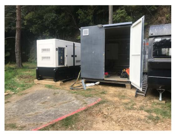
Figure 3 - Generator and control panels in place at the Talisman Mine site
