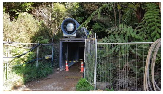
Figure 2 - Main Fan in position above the airlock
