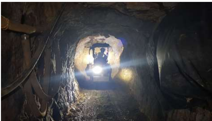
Figure 1 – Cleaning out BM37 Cross-cut
