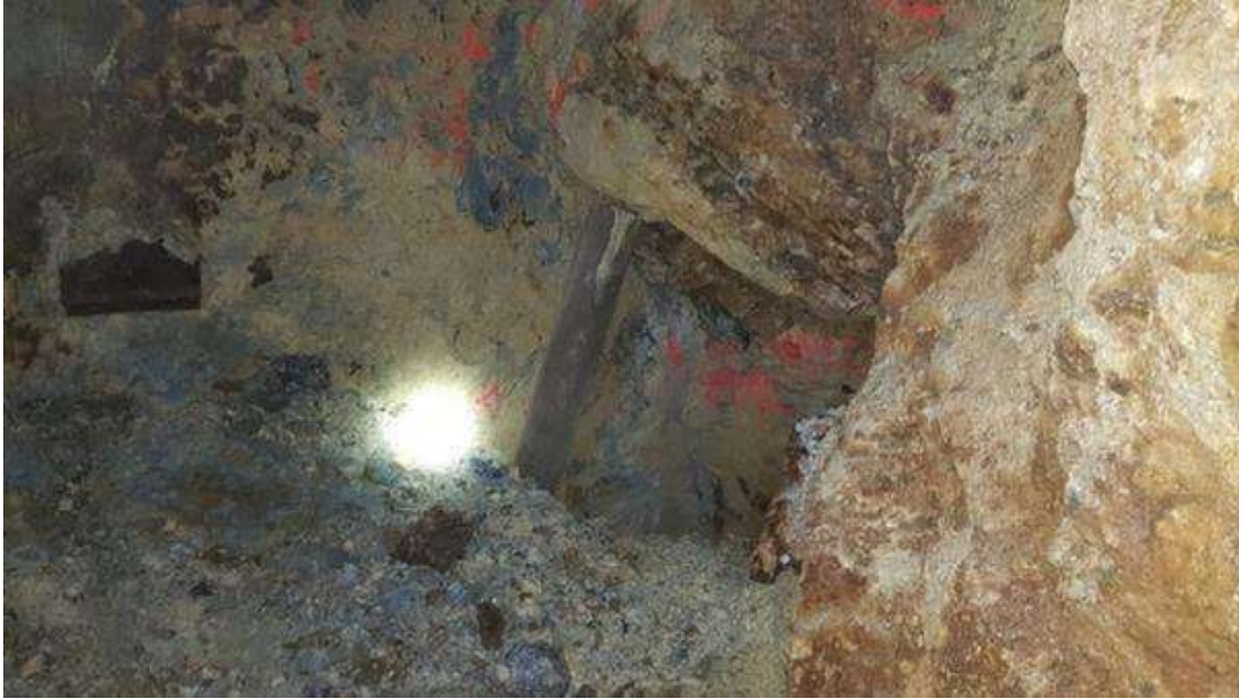
Figure 4 - Historical support in place below the Dubbo Maria Vein exposure
