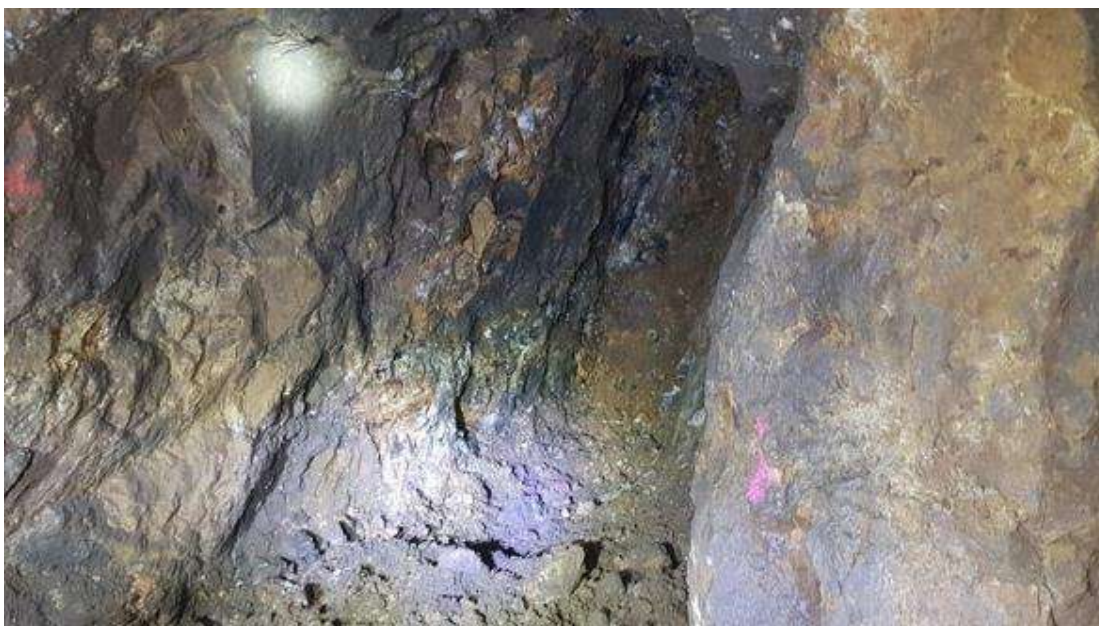
Figure 8 - the face of the Mystery Drive showing the extension of the vein before sidewall waste is removed
